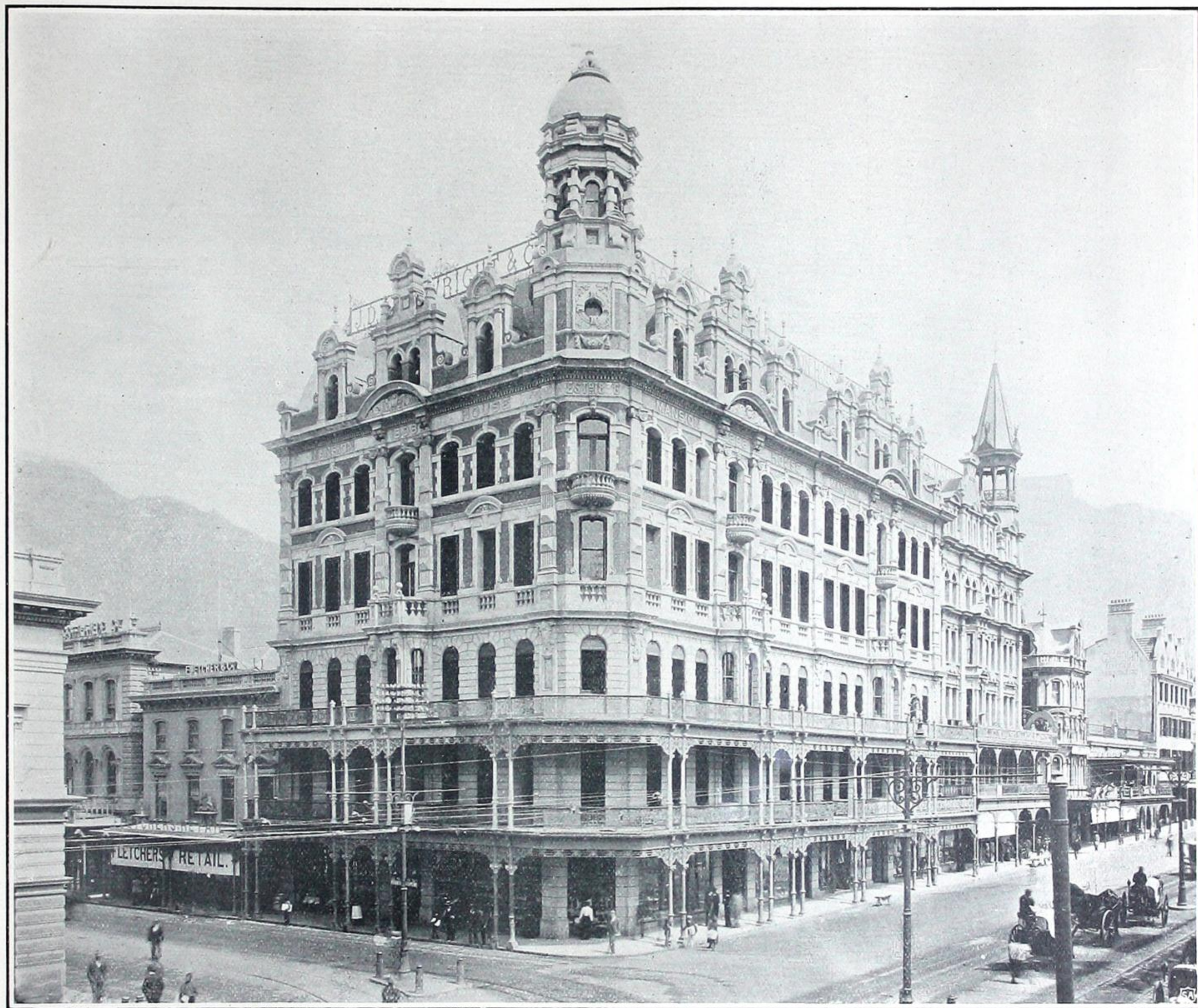
Fig. 194. —Mansion House, Cape Town, South Africa, In which our Embossed Metal Ceilings are used throughout.
